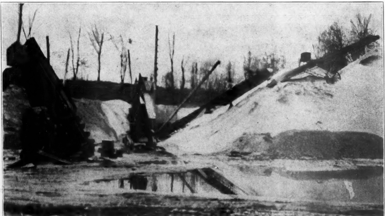
Hartford Yard. Unloading Point in Background and Portable Conveyors Used to Make Piles of Surplus
